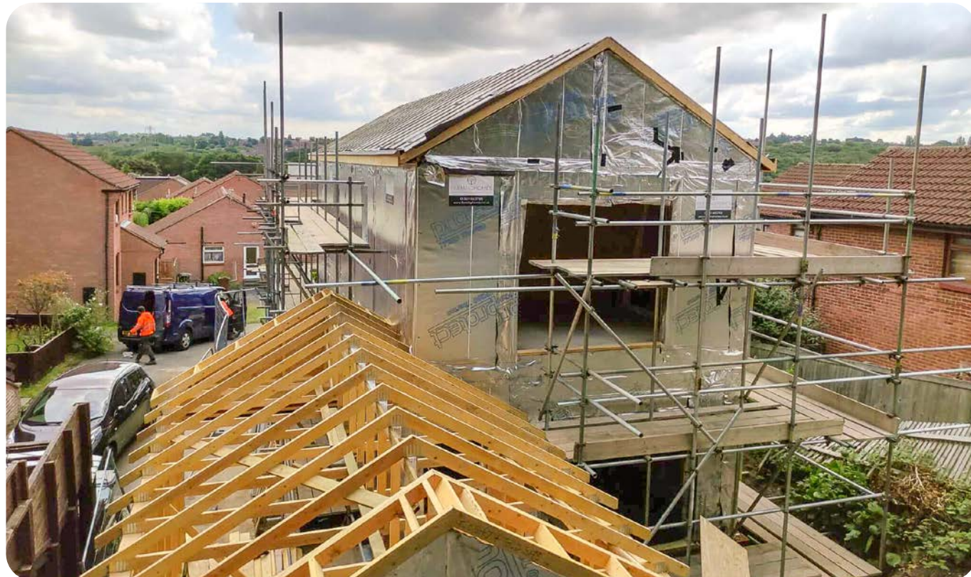
A new self-build home under construction
